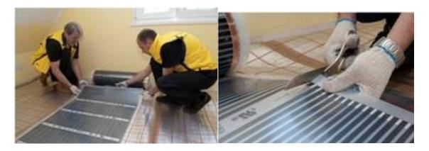
The heating film can be butted together but cannot be overlapped at any time.
