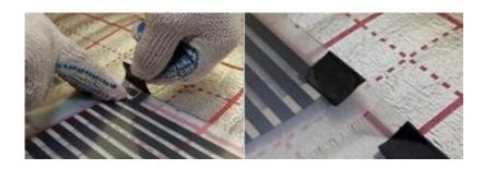
8. Once the underfloor heating mats have been laid and fixed in place over the floor the connection tails should be run back to the underfloor heating thermostat or junction box location. The diagram below shows the two ways underfloor heating mats can be connected back to the underfloor heating thermostat. (Underfloor heating mats must always be connected in parallel never in series).
