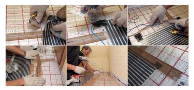
11. Once the underfloor heating film have been laid and fixed in place the vapor barrier is ready to be laid over the top of all the under floor heating film mats. The vapor barrier must fully cover all under floor heating mats. It is not a necessity to cover the whole floor area only the actual underfloor heating film themselves. If necessary the vapor barrier can be taped around the edges to hold it in place.
