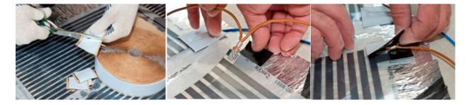
f) In the same way, use the mastic tape to cover all of the bare ends of each copper strip that do not have wire connections.
