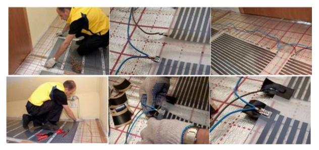
The connection ends and cold tails can be pressed into the underfloor insulation by scoring the underfloor insulation and firmly pressing the tails /ends into the scored underfloor insulation. It
