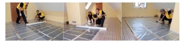
An electrical test of the adjusted heating film must be carried out by an electrician. All mats must be connected in parallel.
